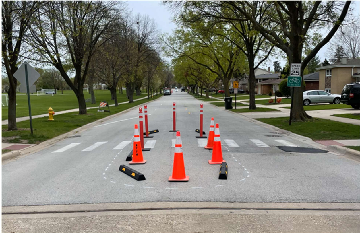
Example Temporary Median Island Installed on William Street
